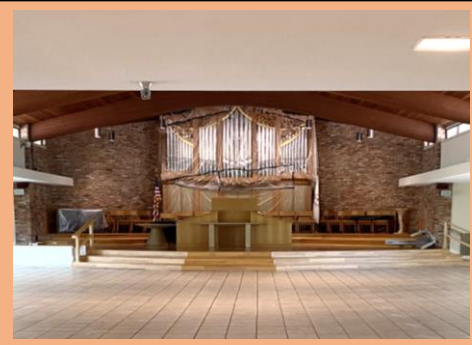
Piano Removed; Organ Pipes Covered, Ready for Demo
