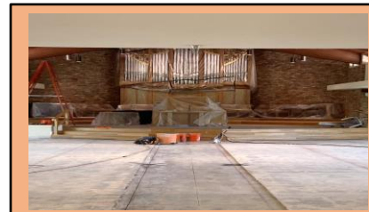
T-Loop Installation
